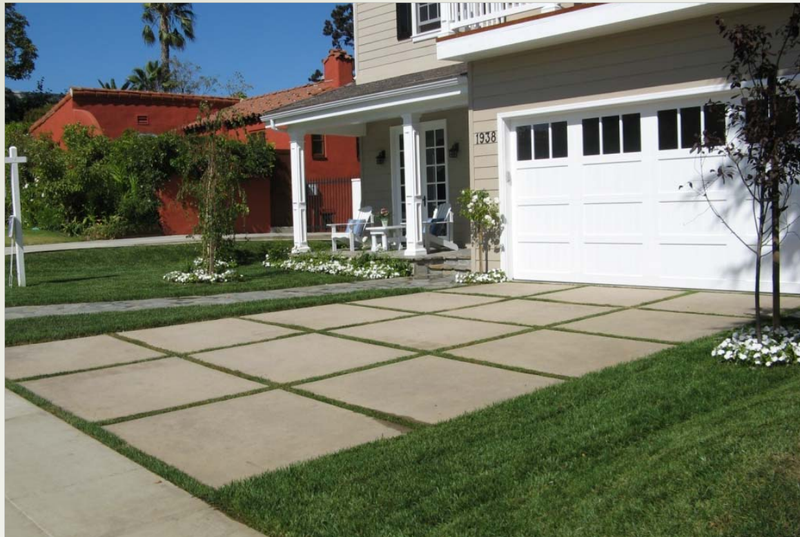
West L.A. driveway with grass to increase permeability
